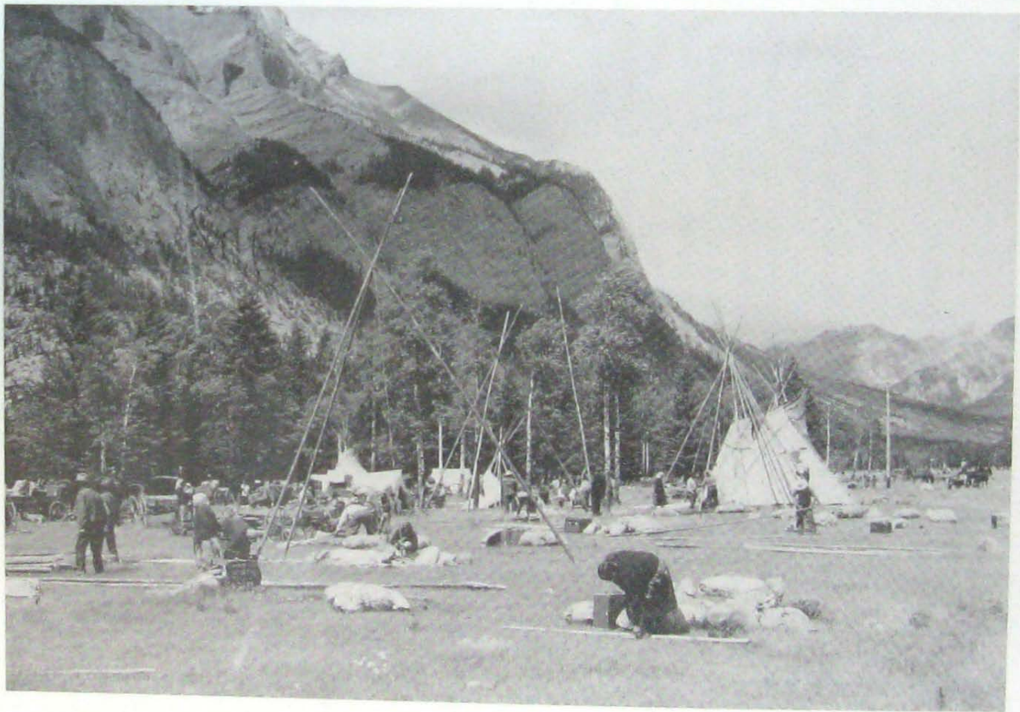
Plate 18: Stony Indian women constructing tipis at Cascade Park, site of the Indian village, 1948. Basic three-pole foundation is shown. Photographed by Fern Gully. Source: Fern Gully.
