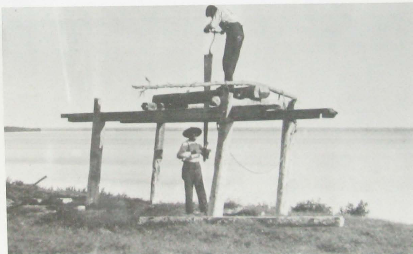
Plate 22: "Two Men Sawing Planks off a Log, North-Western Saskatchewan, 1908-9." [F.J.P. Crean Album, Saskatchewan Archives Board]
